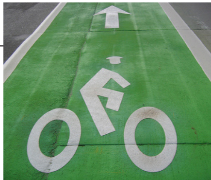
Painting for bike lanes (full lane or mixing zones only) Figure B.1.t
