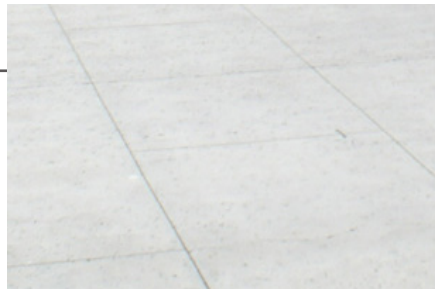
Concrete Paving (Figure B.1.r)
